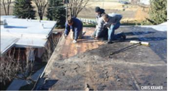
Roofing company employees work to repair damage to the UCA girls' dorm after the windstorm sheared the flat roofing.
